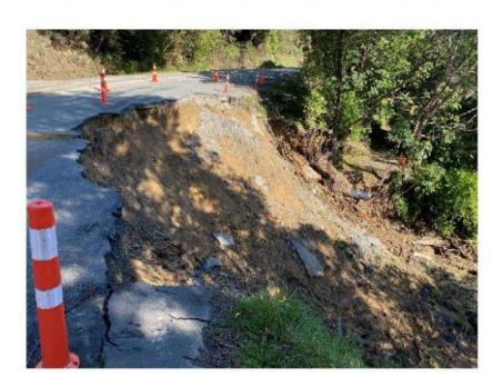
A repair of a significant underslip that potentially requires the road to be retreated into the hill by 4m.
